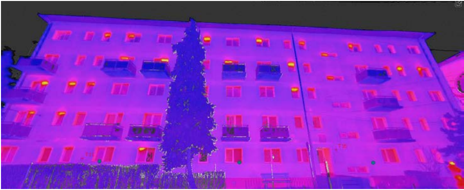
Figure 1. Facade with temperature attributes obtained from final processing
